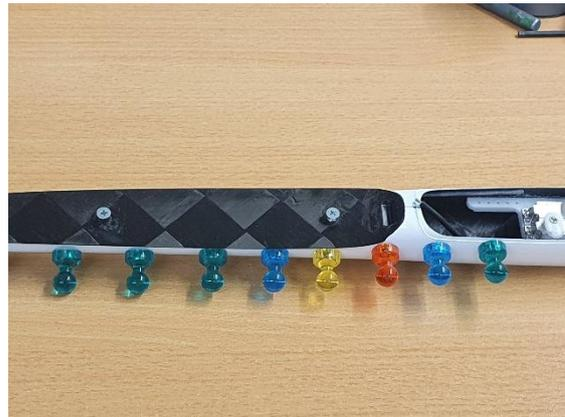
Then apply thin CA to the outer part of the tube and let the model rest vertically while curing.
